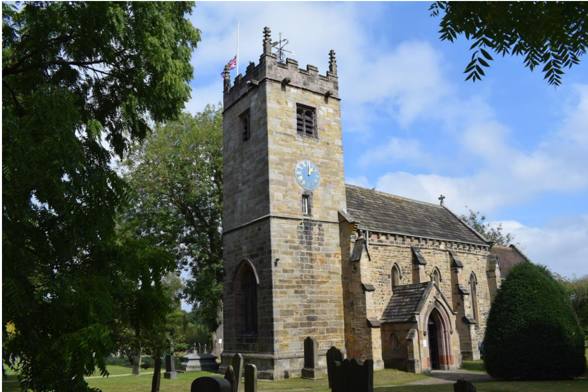
Figure 1 - St Oswald's Church, Collingham, West Yorkshire
